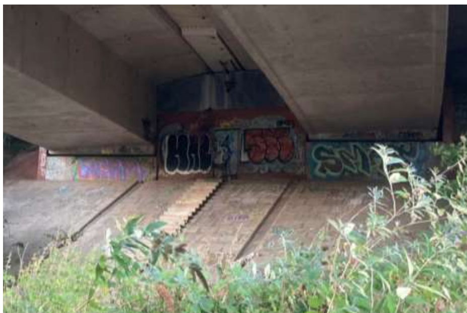
Photograph 5: A4055 Flyover eastern access tunnel
