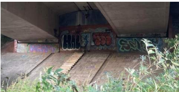
Figure 1.11 Access Tunnel entry of A4055 flyover (TN4 Figure 4)
