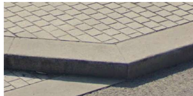
Kerb Type 1.: Granite Road Kerb (150mm Raised) Kerb Type 2.: Granite Road Kerb (Flush) Size: 150x200x500mm Colour: Silver grey Finish: Bush hammered Supplier: Stonepave or similar approved
