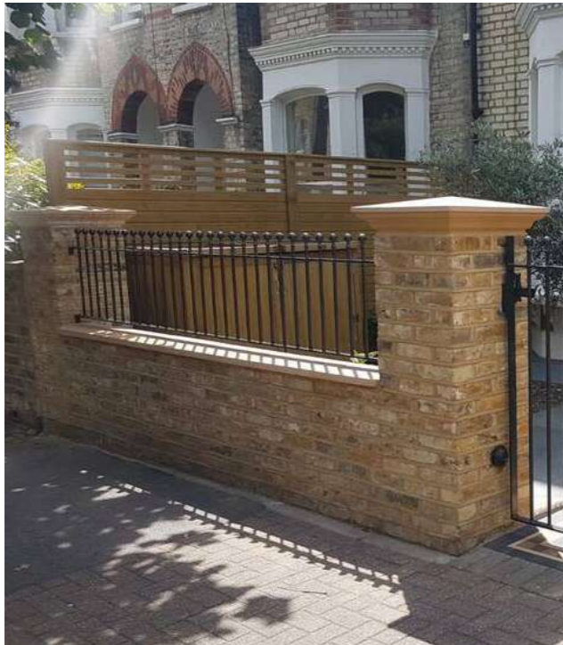
Low wall and metal railing to form communal terrace.
