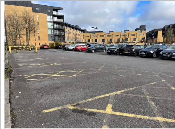
Photo 1: Plot 1 – View south-east across car park towards residential properties
